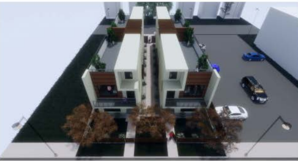
Figure 24 – View from Churchill Avenue
